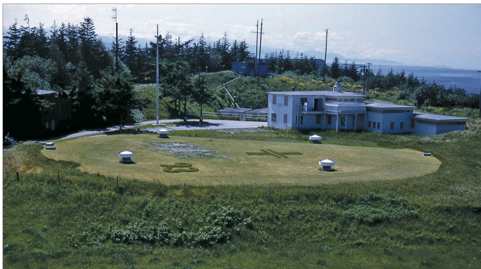
This view looks westerly up the Strait of Juan de Fuca at the original Coast Artillery fire control building. The Harbor Entrance Control Post (with stairs) is in the center background; it's the tallest point on Artillery Hill. The rooftop of the 1908 Ready Barracks (where soldiers on duty at an Artillery Hill gun battery, for example, would stay), located in a depression below the HECP, is also visible. Washington State Parks burned/demolished all these wooden structures in the early 1970s. -Photo from Coast Artillery Museum Collection
