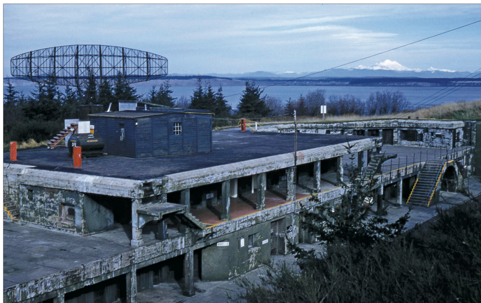
Here's a view of the long range radar unit mounted on a cinderblock structure built atop Battery Benson (the 10-inch cannons had been removed in 1944). All that remains today from this photo is the main cinderblock building. -Photo from Coast Artillery Museum Collection
